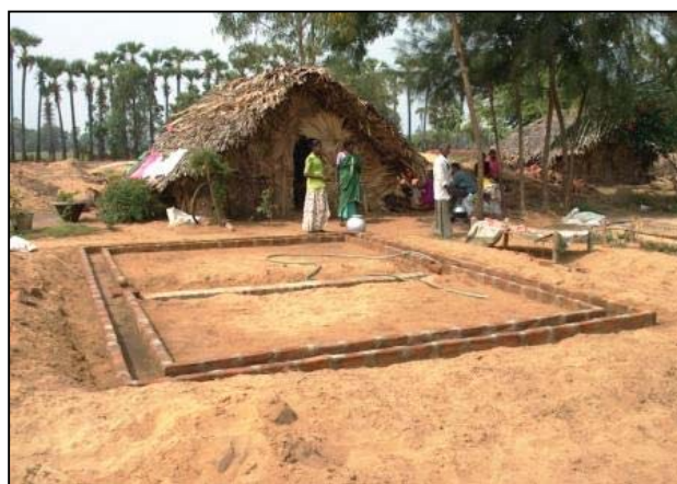
Foundations for Tsunami Relief House
