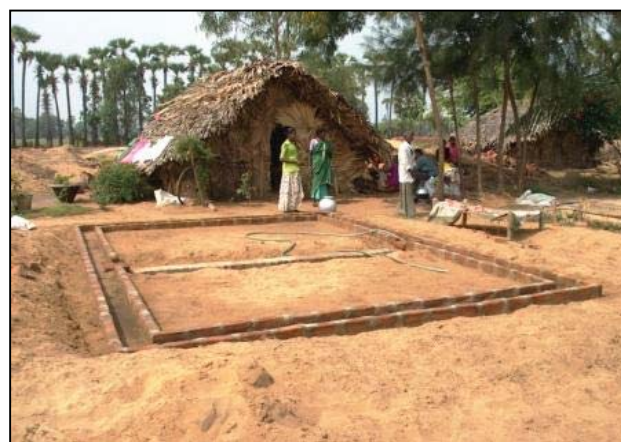
Foundations for Tsunami Relief House
